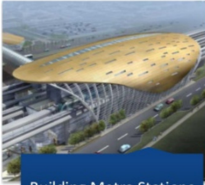
Building Metro Stations
