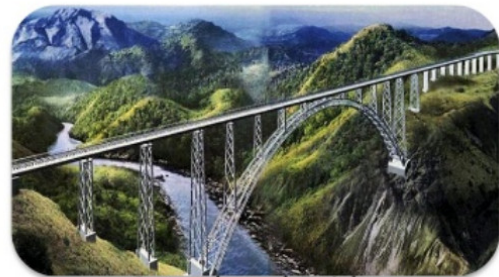
Completed Bridge – Objective achieved
