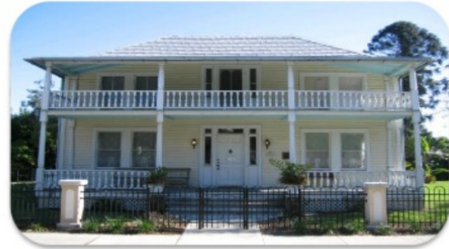
Constructed House – Objective achieved
