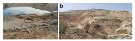
Figuer 6: Landslides in the lower FHS: a) 2013 when a major collapse took place, immediately east of the dam, b) just west of the Mujib Dam when it started during 2011.
